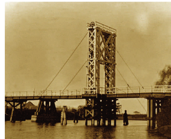
The original Kinchela Bridge.
